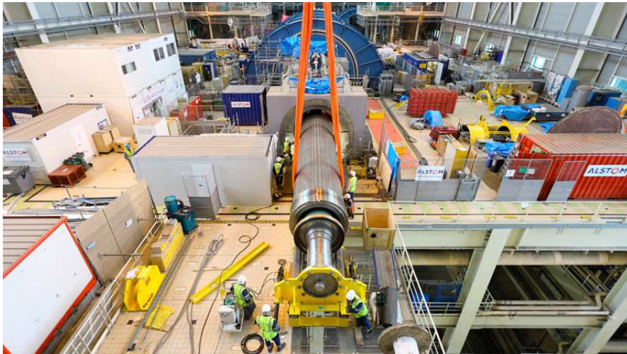
FIGURE 1.6 – Rotor EPR Flamanville
